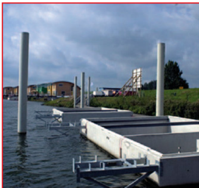
A floating concrete basement provides buoyancy and additional living space.
